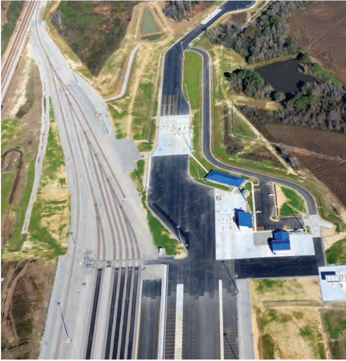
Terminal north lead looking north
